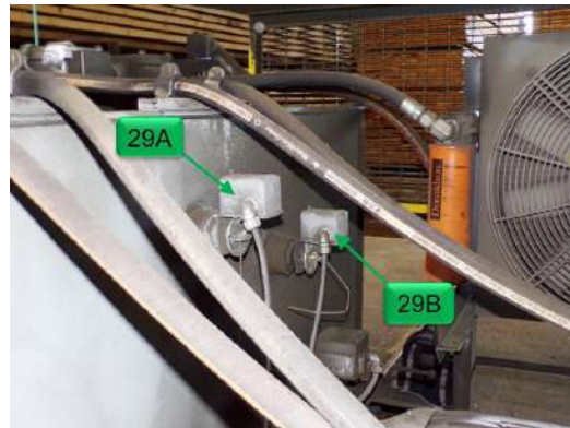
No. 29A & 29B Level Switches
