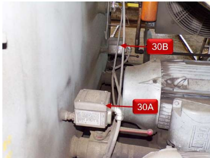
No. 30A & 30B Temperature Switches
