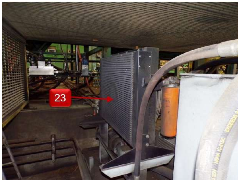
No. 23 Heat Exchanger
